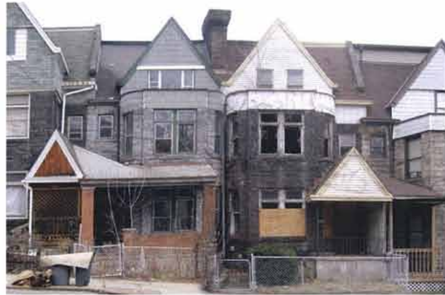
abandoned buildings in very poor condition...
