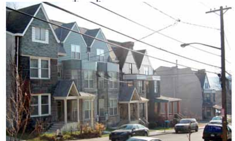
• Removed stone facades of 218 and 220, constructed new units, rebuilt stone facade
