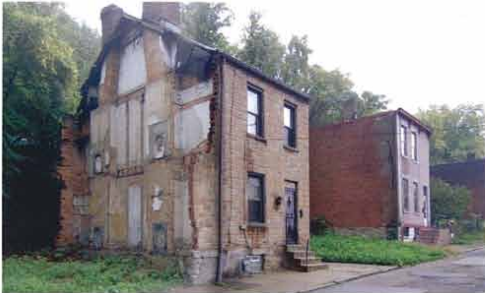
gaps and deteriorated buildings on Wick...
