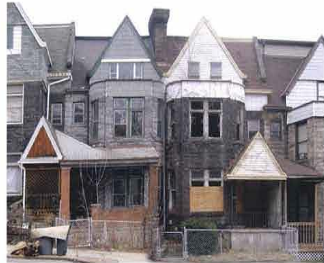
abandoned buildings in very poor condition...
