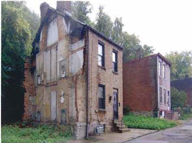
gaps and deteriorated buildings on Wick...
