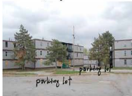
parking lot parking lot no public-oriented green space
