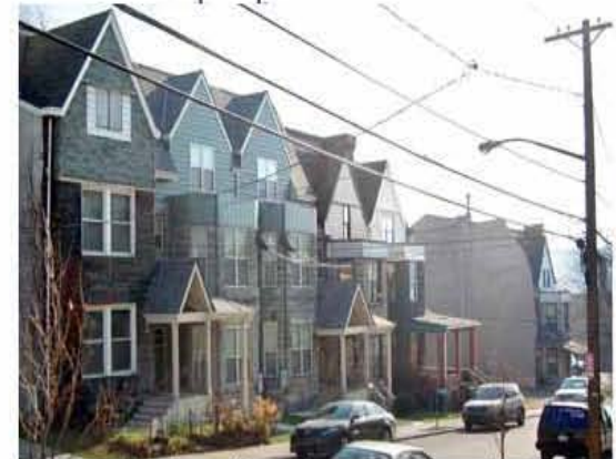
• Removed stone facades of 218 and 220, constructed new units, rebuilt stone facade
