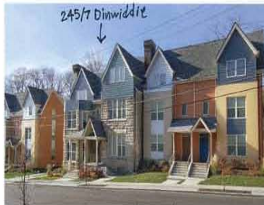
• Historic building integrated
