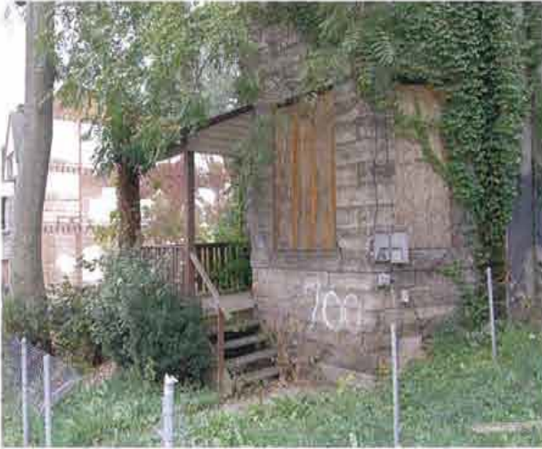
many abandoned buildings...
