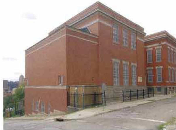
existing Auditorium (below) and Gym (above) of historic Miller School.
