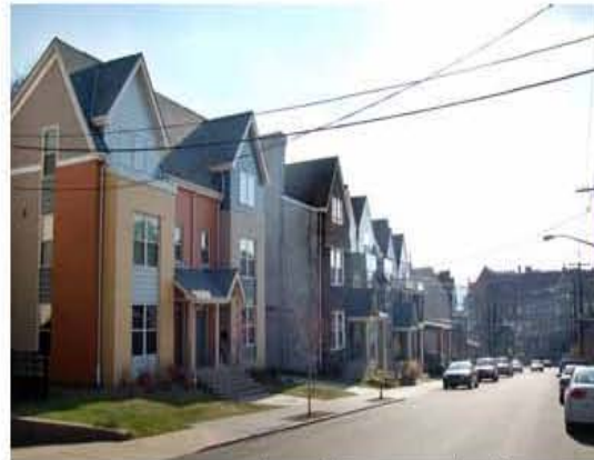
• Density reestablished on east side
